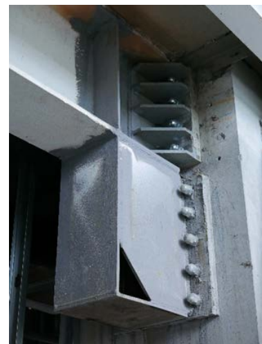
Fig. 4. The connection of the strengthening scheme
