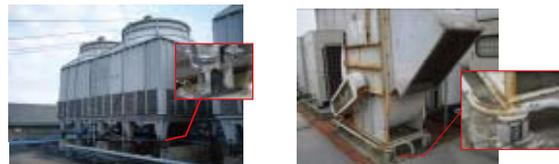
Figure 2. Leakage damage of a spring isolated cooling tower after Hwa-Lien earthquake
