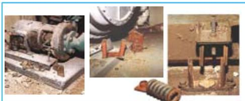
Fig. 1 Damaged vibration isolation devices due to earthquake.
