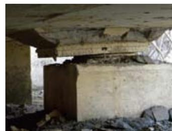
Figure 4: Displacement and damage to supports
