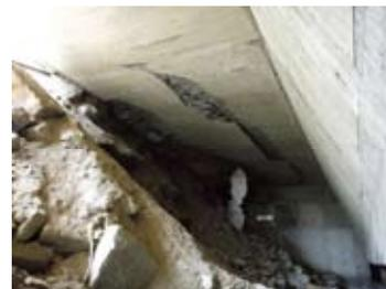
Figure 3: Damage to the outer box girder
