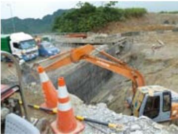
Figure 5: Repair of the abutment back wall
