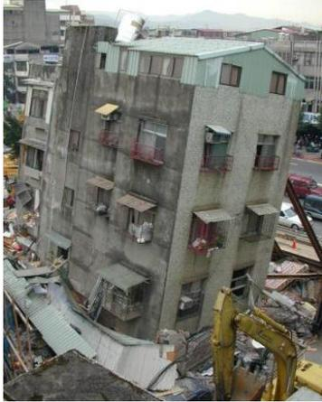
Fig. 1. Bottom two stories of a five-story apartment after collapse in a major earthquake.
